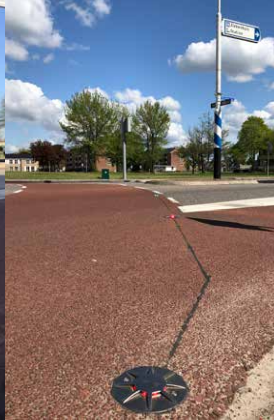
When the ThermiCam units detect the heat signatures of vehicles and cyclists, they activate in-road LED warning signals that guide cyclists towards the parallel bike lane.
